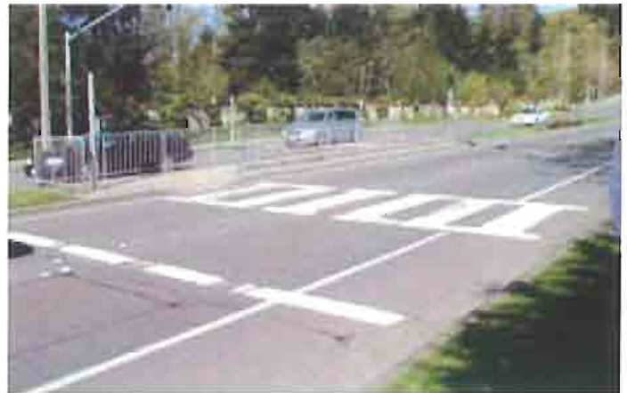
Advanced stop bar and ladder striping enhance visibility for pedestrians.
